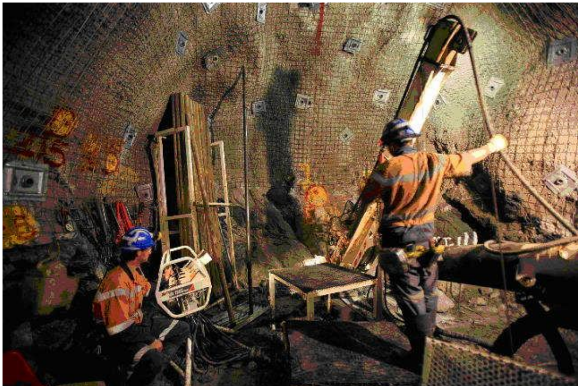
Figure 10: Underground Drilling at the Lanfranchi Nickel Mine
